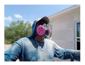
Common sense should be used when cutting panels. It is a good idea to orient the cutting area so prevailing wind blows away from the project and other workers. Likewise, the cutter should have the wind at his back or side to help push dust away from him.
