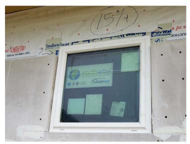
Once windows are installed the nail flange is flashed to the adjoining weather barrier. First cut the head piece diagonally away from the top corners and fold up. Jambs are taped first, then the head. Flashing tape should cover the fasteners and effectively seal the nail flange to the weather barrier. Fold the head piece down over the head flashing and tape the cut ends to the weather barrier.
