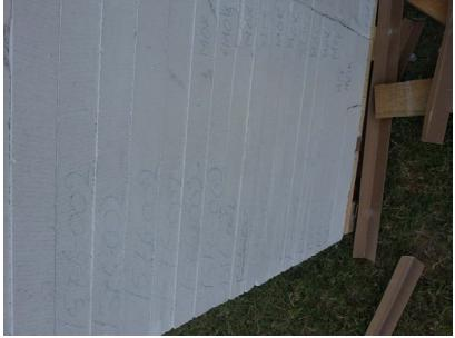
Apply pressure and bend the panel so the panel breaks on the uncut side following the cuts on the other side.
