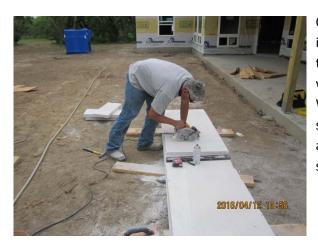
One of the components in manufacturing AAC panels is silica, a known carcinogen. Silica is present in most types of cement products. All powdered cements warn against breathing cement dust during mixing. When cutting AAC panels, silica dust is created by the saw blade cutting into the panel. Because hand tools are used the worker is very close to the source of silica dust.
